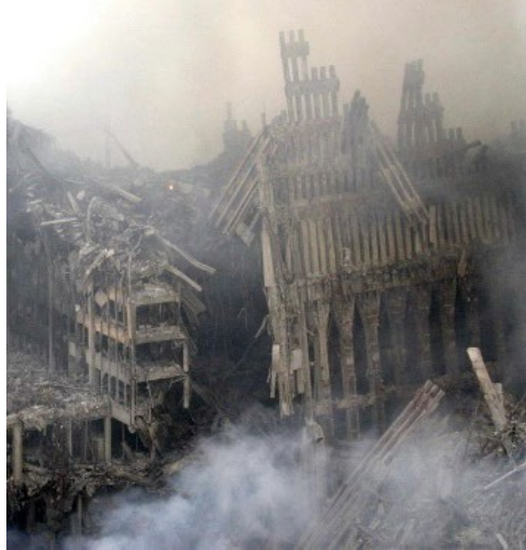
Figure 19: The destruction of the World Trade Towers on 9/11/2001 is similar to the type of damage that might be seen in the SDZ.
