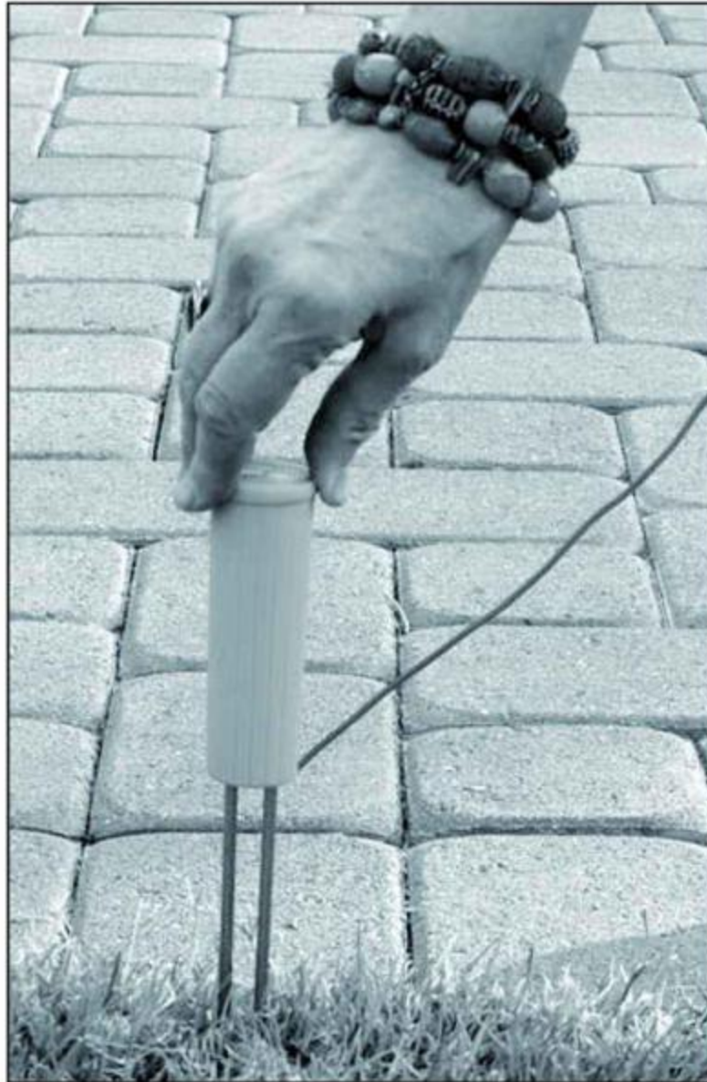
Figure A-1. Placing ground rod in Earth.
